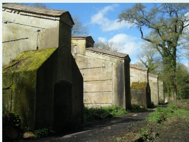
1880s steam incorporating mills, where underfloor gear rooms and blast-proof walls still remain
