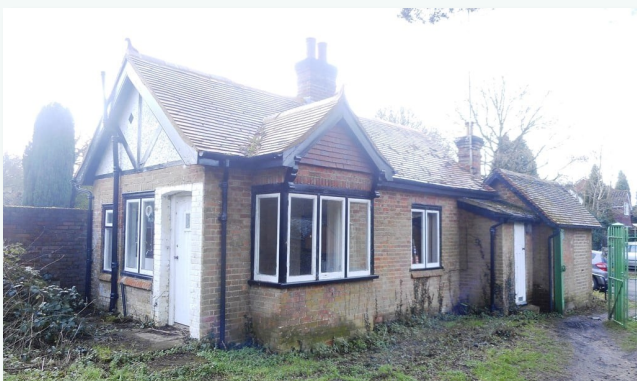
West Lodge gate house, where workers would check in for materials that might cause a spark
