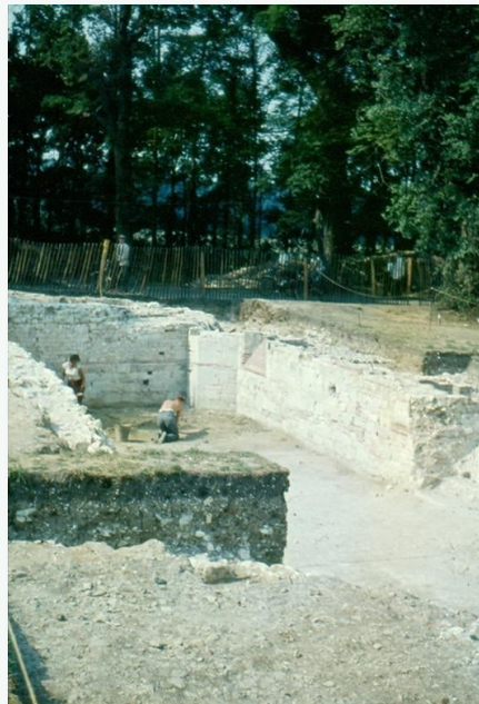
Excavation of wine cellar (Steve Nelson)
