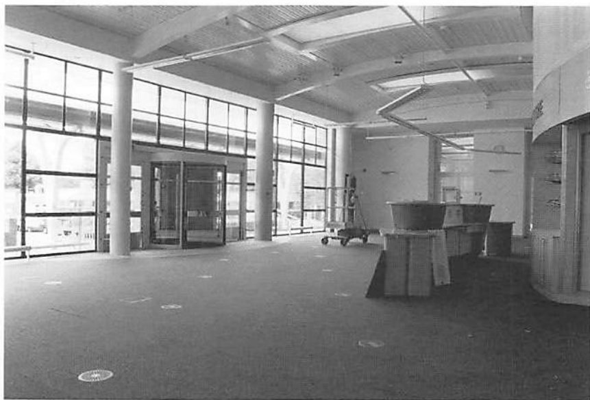
Fig. 3. Surrey History Centre: Entrance Foyer during the fitting-out process.
