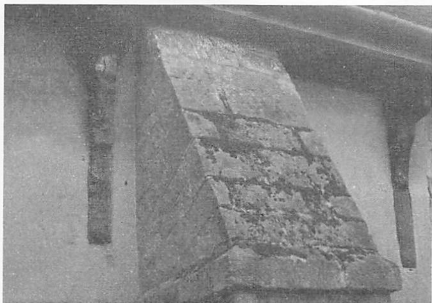
2. Timbers on the South wall of the Chancel at Witley Church
