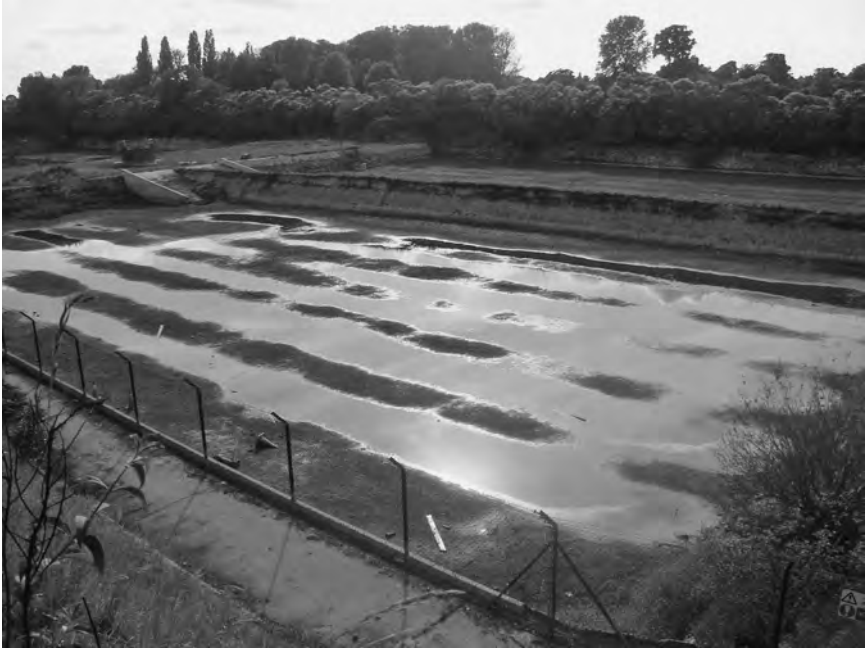
Figure 4 One of the filter beds that was drained in 2011. It shows the undulating surface of the beds, which is a result of the large ceramic pipes at the bottom. – Howard Bengé
