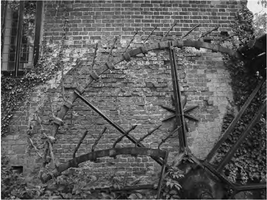
Figure 9 Photograph of the derelict iron waterwheel of the engine house taken in 2010.
