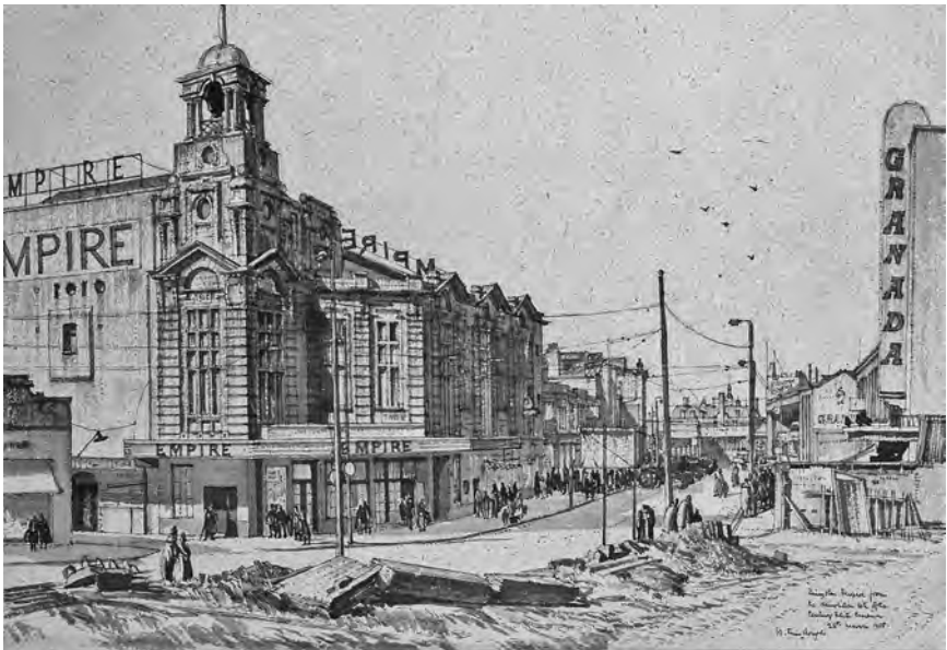
Figure 7 The Empire Theatre and the site of the Elite Cinema in Kingston, 1955 by Wilfred Fairclough ( Brill Collection no.3, reproduced courtesy of Kingston Museum & Heritage Service)
