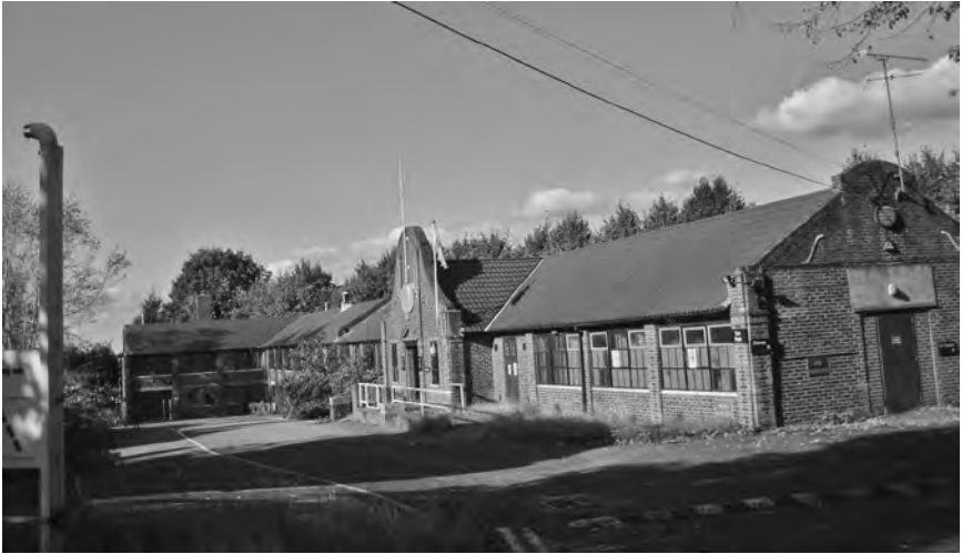
Figure 5 The empty Thermega/Remploy Factory: photographed by the author, 2008
