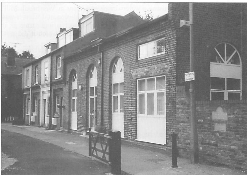
Fig 2 Weybridge's first power station.
