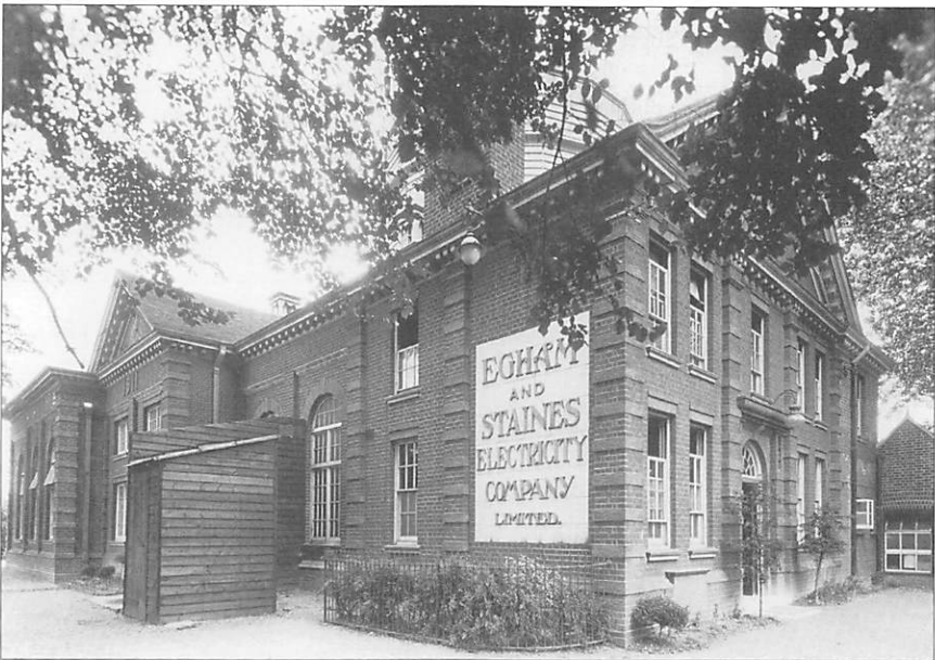
Fig 3 Egham's second power station. Courtesy of Amberley Working Museum.
