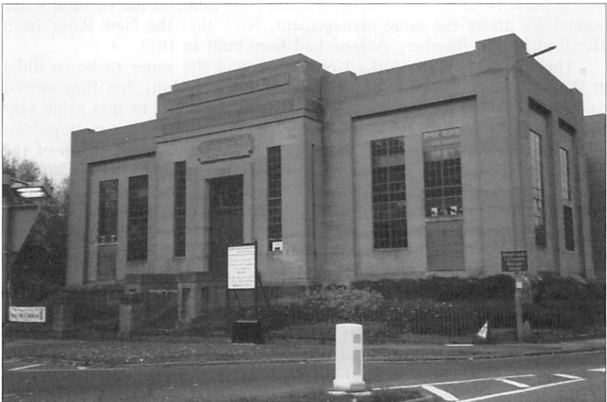
Fig 4 The East Surrey Water Company’s pumping station, Leatherhead.
