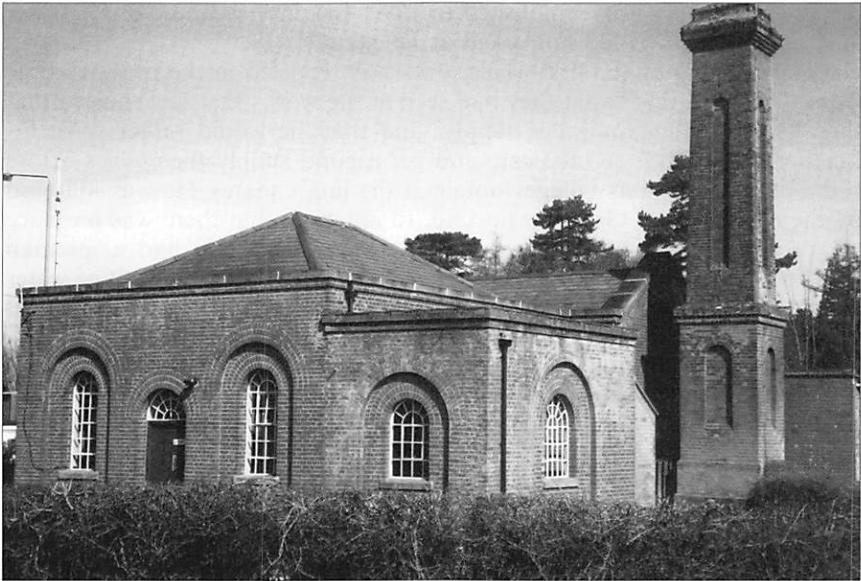
Fig 5 Woking and District Water Company's pumping station, Horsley.
