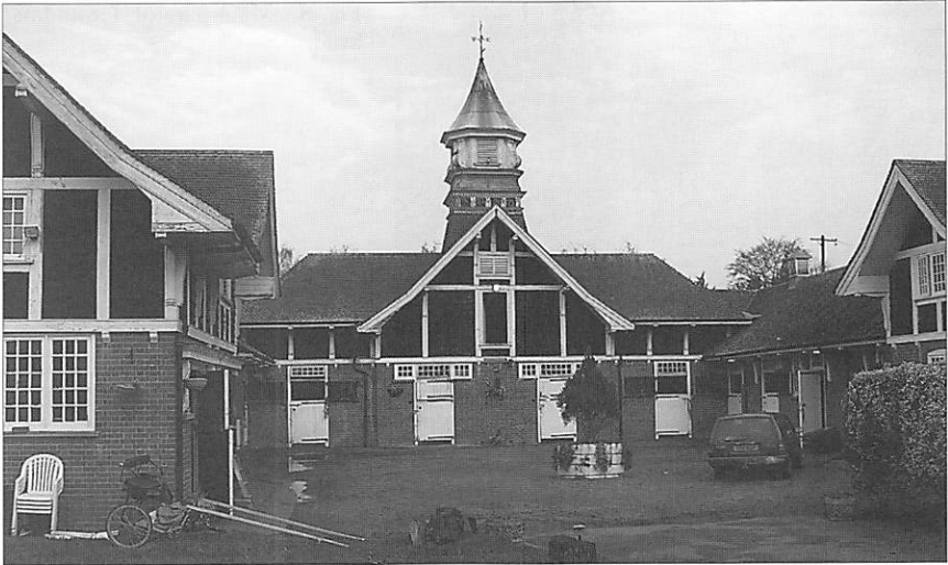
Fig. 6 South elevation of Cicero Stables.
