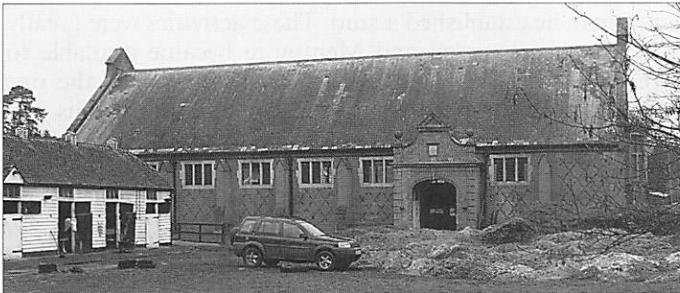
Fig. 1 South elevation of Riding School.
