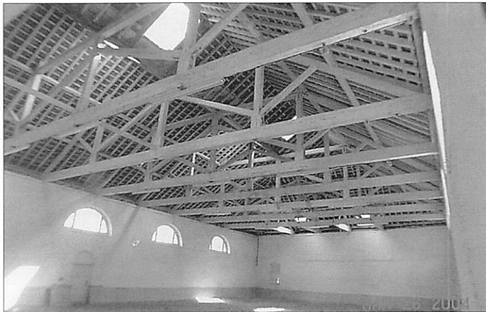
Fig. 5 Roof structure of Firle Place riding school.
