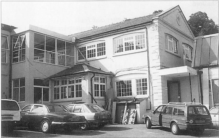
Fig. 1 The Langham Factory, Godalming, in 1990. (Photograph by Glenys Crocker.)
