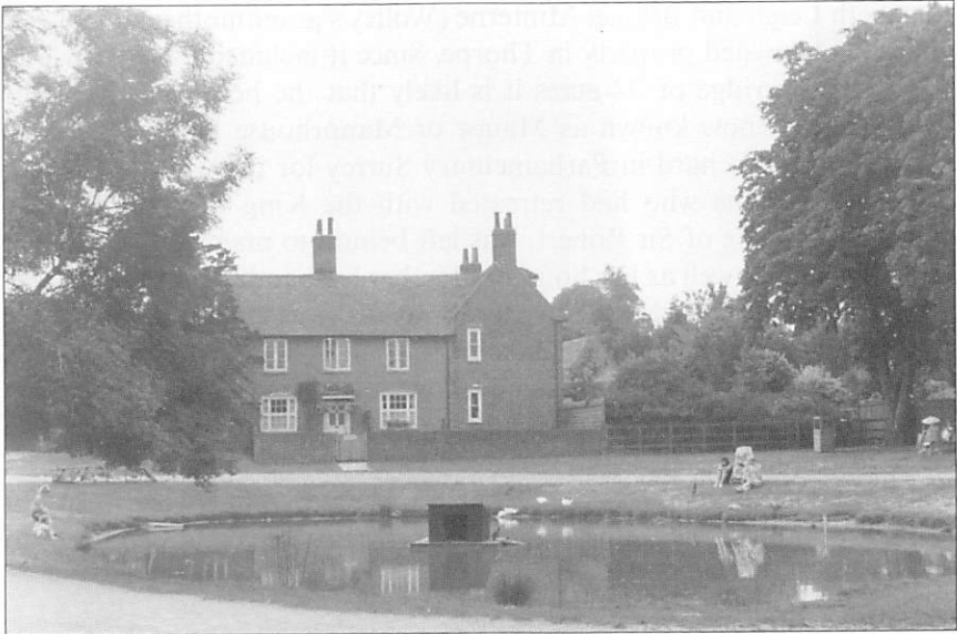
Fig.4 Manorhouse Farm, Coldharbour Lane, Thorpe: The left-hand side of the farmhouse is a typical lobby entry, central chimney building of the early 17th century. It would have been new when the Perry family were living there in 1643. (Photograph 1990 by the late Desmond Mills.)
