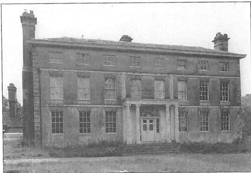
Fig. 4 Front elevation of Shalford House in 1967 from a photograph held by the NMR.
