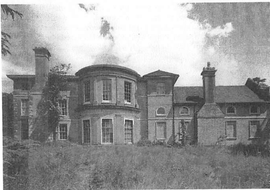
Fig. 7 The northern wing of Shalford House showing (from left to right) the original house of 1608-10 with exterior alterations of 1797, the bay window which was added as a single storey in 1829 and the extensive additions of 1875. From a photograph held by the NMR.
