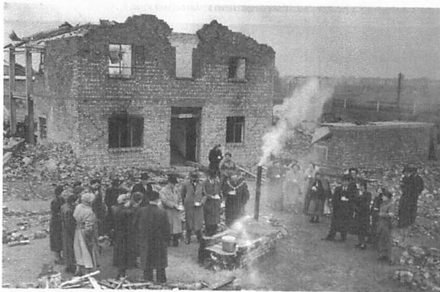
Fig. 6. Civil Defence emergency feeding demonstration at Epsom in the presence of the mayor and mayoress, 1954. The cooker was improvised on site from bricks, a metal sheet to serve as a hot plate, an old iron grid for fire box and drainpipe sections as a chimney. A 'pug' of earth and water was mixed to act as cement. [GMR 5380/1/10(4)]
