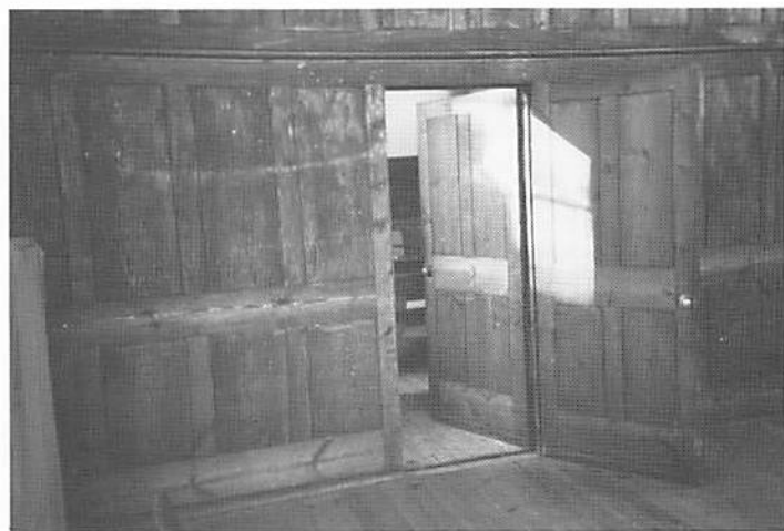
Fig. 5. Dorking Quaker Meeting House. Double doors through the lower partition.
