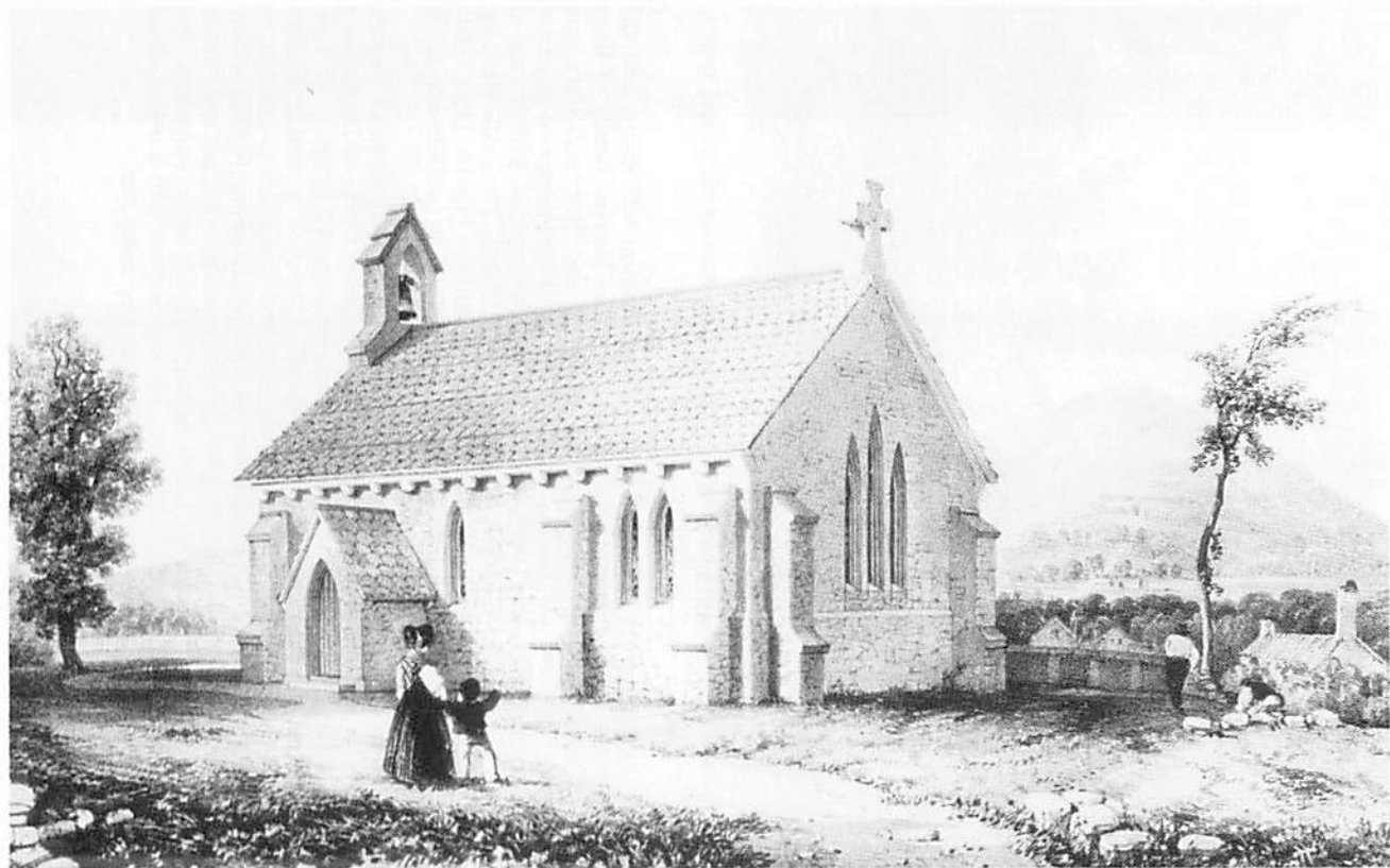
Fig. 2. North Holmwood Church, by J.B. Watson, Architect.
