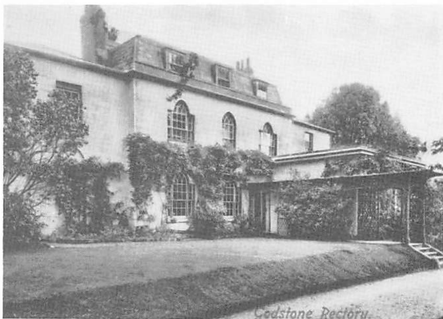
Fig. 5. Godstone Rectory about 1910. Sometime in the nineteenth century an additional storey was added to accommodate the rectors' large families.
