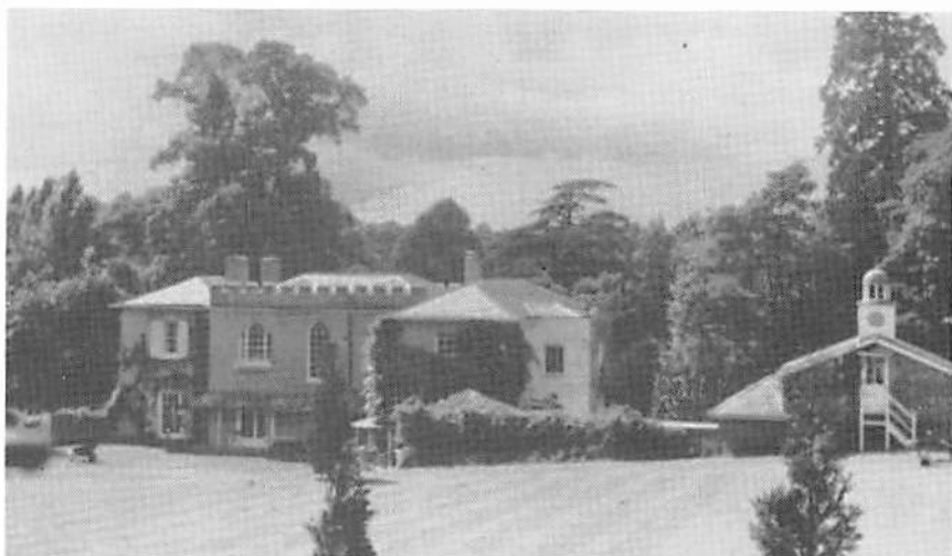
Fig. 6. Godstone Rectory in 1990. In 1944 the rectory and the glebe land were sold into private hands and The Homestead in Bulbeggars Lane purchased for use as a parsonage house, a use that continues to this day. In the fifties the old rectory, now called Glebe House , was restored to its two-storey origins and crenellations substituted for the rather bleak parapet.
