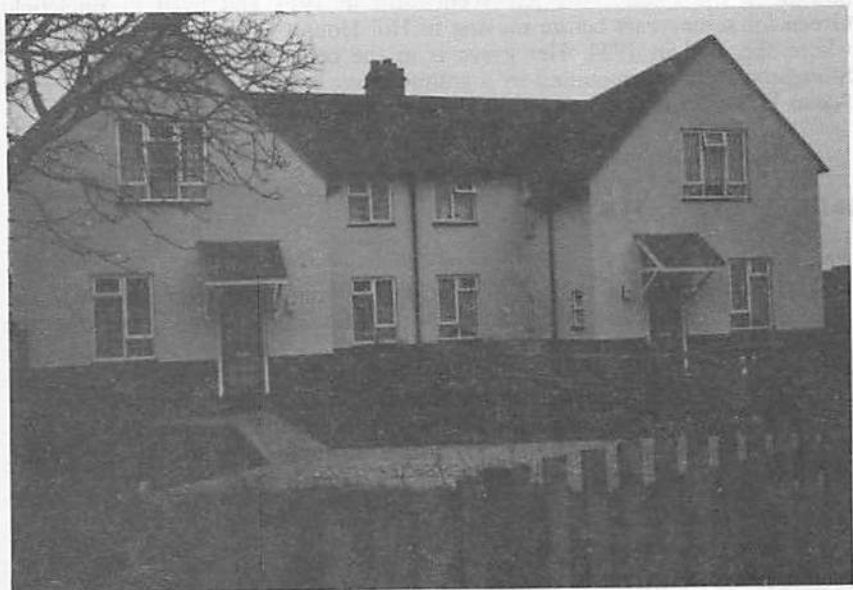
Fig. 5. Modernised two-storey houses at Shepherd's Hill.
