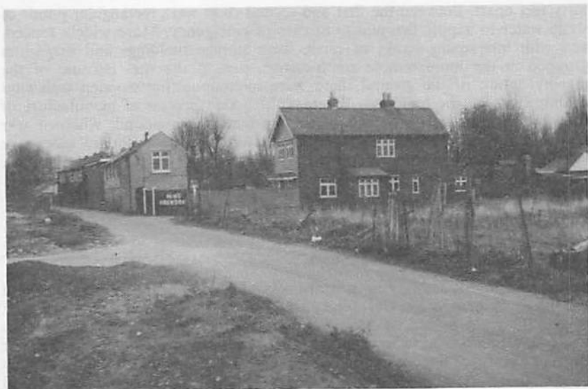
Fig. 8. Pain's Firework Factory from Firework Lane, Mitcham, photographed in April 1966, after production had ceased. The derelict land in the foreground is part of the former market gardens of F. & G. Mizen.
