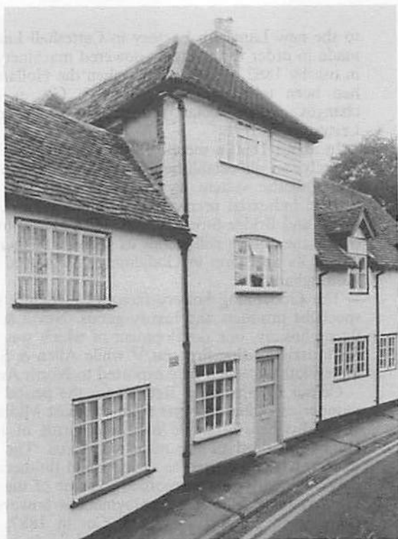
Fig. 6. Front View of 22 Mint Street. The top storey of the rear workshop was later extended over the front of the house.
