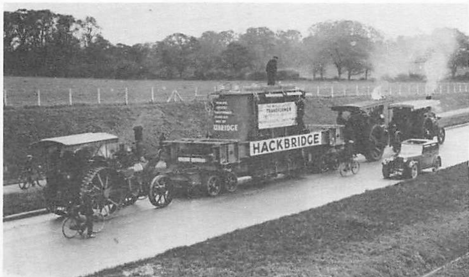
Fig. 2. The second transformer on the Kingston By-pass in April 1933 (from the collection of Mr. Alan Martin).
