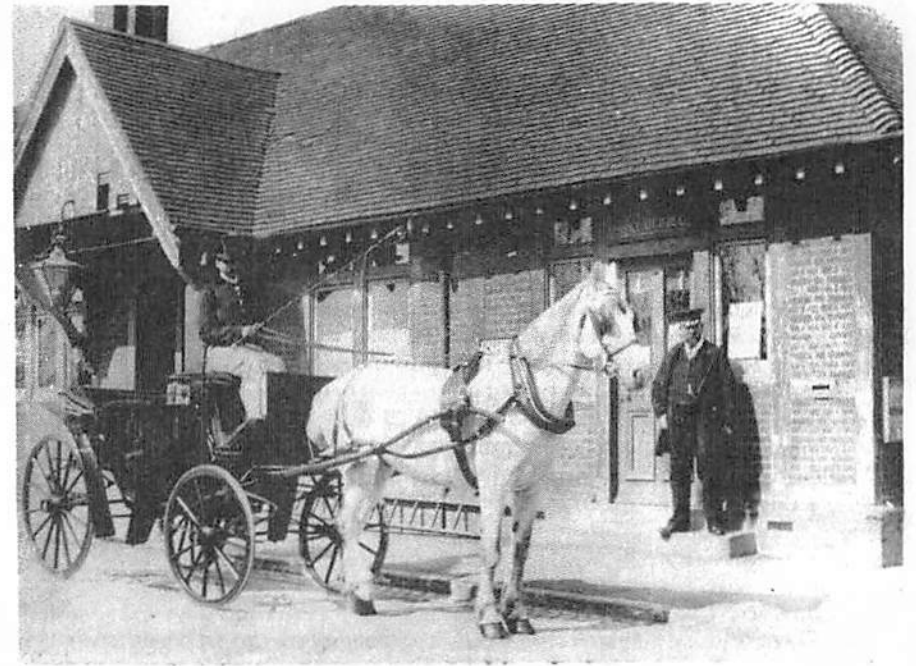
Fig. 4. South Nutfield Station (photograph believed to have been taken about 1920).
