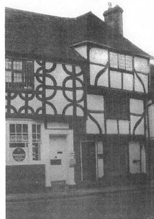
Fig. 4. Houses behind the Town Hall at Godalming. That on the left was the house of a prosperous clothier, who could afford ornate timberwork. That on the right, turned end-on to the street, is a typical townhouse.
