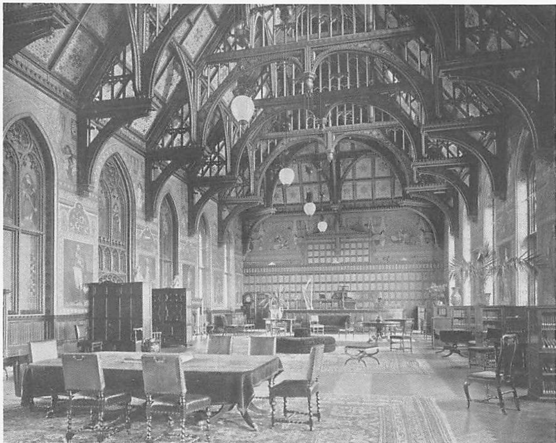
Fig. 3. The Sanatorium, showing the recreation hall, c.1900.
