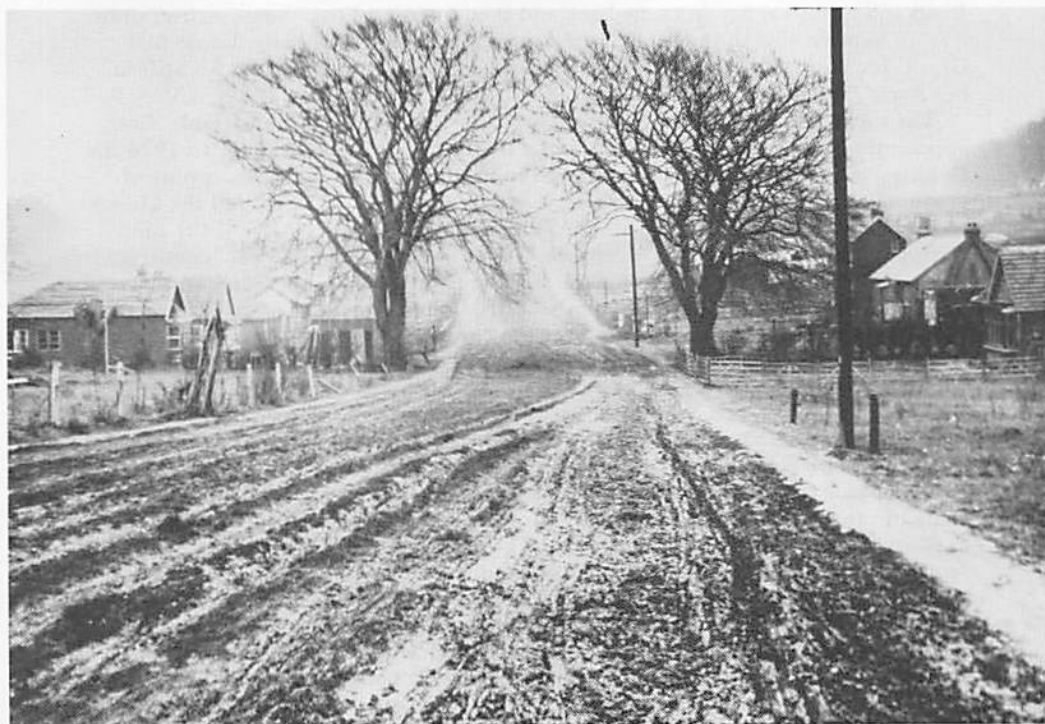
Fig. 5. Dowlans Road, Great Bookham, looking eastward, 10 February 1930. The house on the left had been unfinished for four years.
