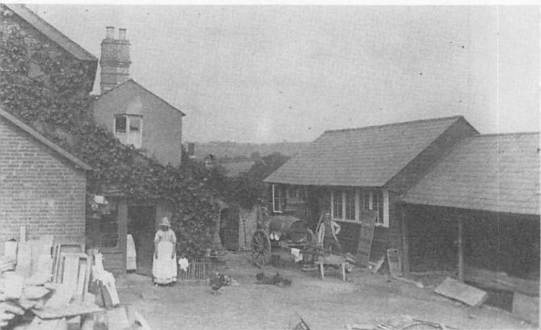
6. Wardle's (Builder's) Yard, Lower Street, Haslemere, 18 August 1886.
