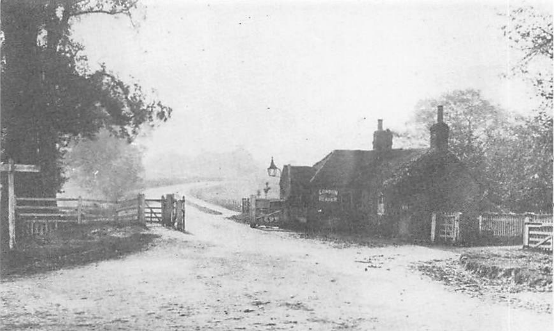
5. Toll gate, Woodhatch, Reigate, looking south ? in 1860s.
