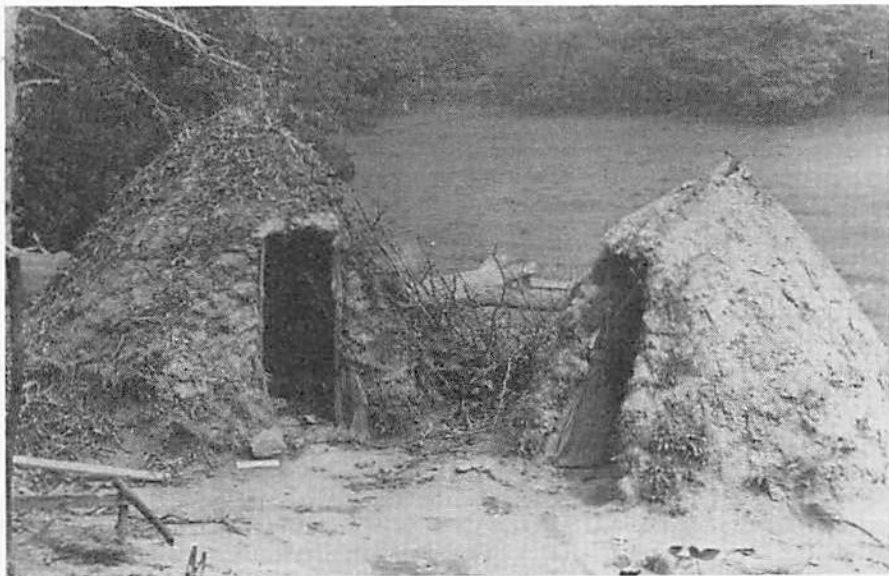
13. Charcoal burners' huts, The Chase, Haslemere. These huts accommodated a family of six. The huts had a framework of wood, and were covered with sods. The measure (on ground—white) is one foot. 16 August 1910
