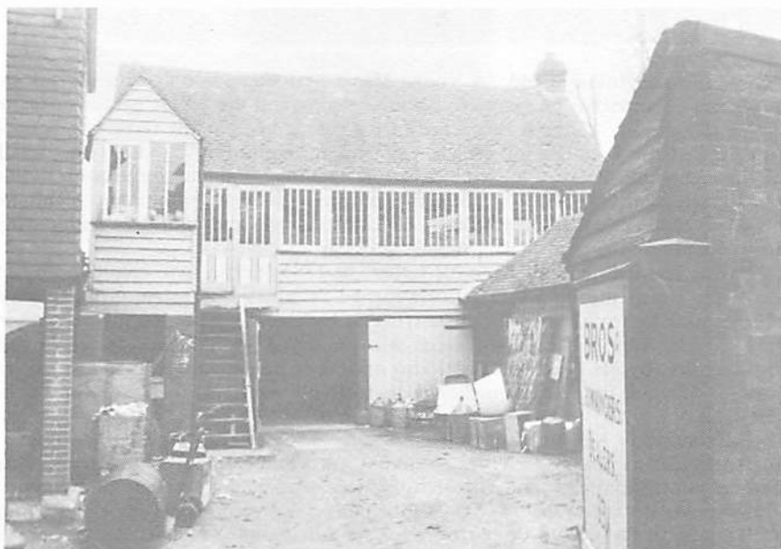
1. Former Carpenters shop, Knockhundred Row, Midhurst
