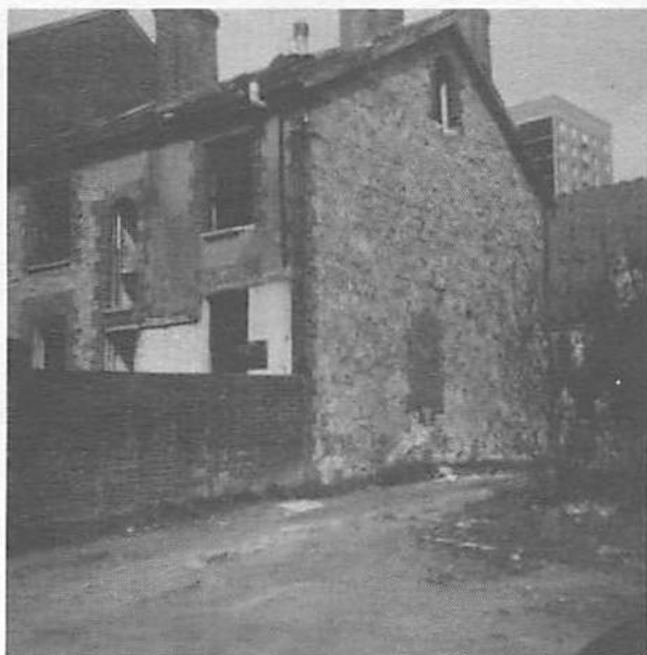
Exterior of 106, showing window and letterbox in east wall.
