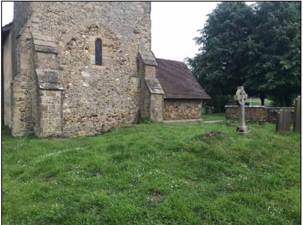
Figure 1: The site of the 1975 excavation west of the tower. The top of the reconstructed Phase 2 northern wall foundation can be seen at the foot of the nearer of the two west-facing buttresses. The bump to its right marks the Haynes vault. On the extreme left of the photograph, the north-west quoin of the probable pre-Conquest nave is visible, although unfortunately covered in render. (Photograph by Rob Briggs, June 2018)
