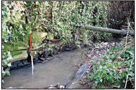
Pipe and brickwork in streambank
