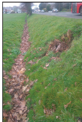
Giiggs Hill, Ditton embankment
