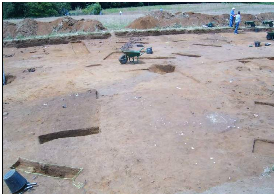
Fig 6 View of part of the lower end of the trench looking west. The location of the villa can just be seen in the left background, showing how close it is to the hilltop site. In the middle ground of the trench the course of the lower curving ditch can be seen heading towards the two figures. The edge of one of the large pits can just be seen to the left (note ladder).
