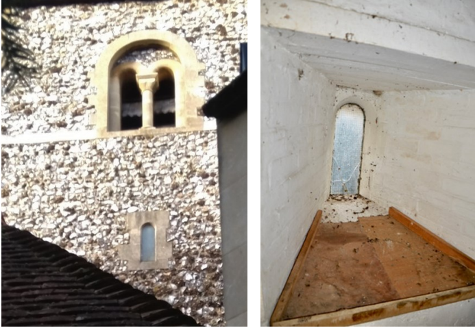
Figs 3 & 4 Former tower west window now on south side
