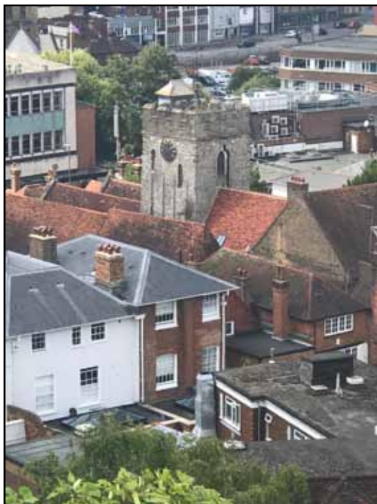
Figure 2: View of St Mary’s church, Guildford. Note the original flint pilasters on the south and east elevations of the tower, beneath later belfry openings and parapet.
