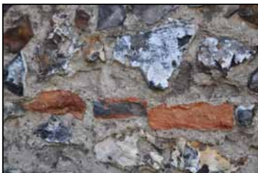
Figure 2: Roman tiles laid above the lowest layer of ferricrete blocks in the north wall of the 12th century nave.
