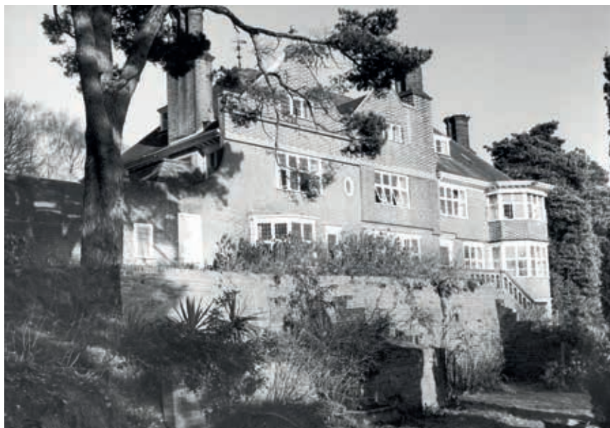
Fig 4: Exterior view of Quartermaine (formerly Stootley Rough School), Farnham Lane, Haslemere, 4 Jan 1965 (SHC ref CC1101/3/75/74)
