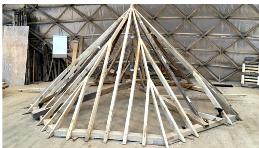
The restored roof structure assembled in the workshop of the grid-shell building
