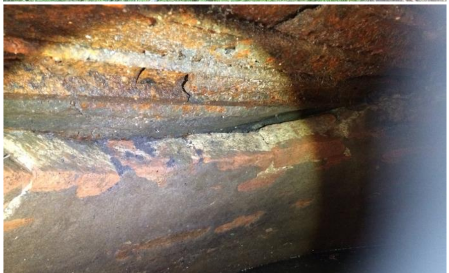
Outside and Inside the Mystery Underground Chamber.
